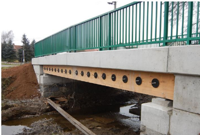
Bark beetle wood bridge, South Bohemia
