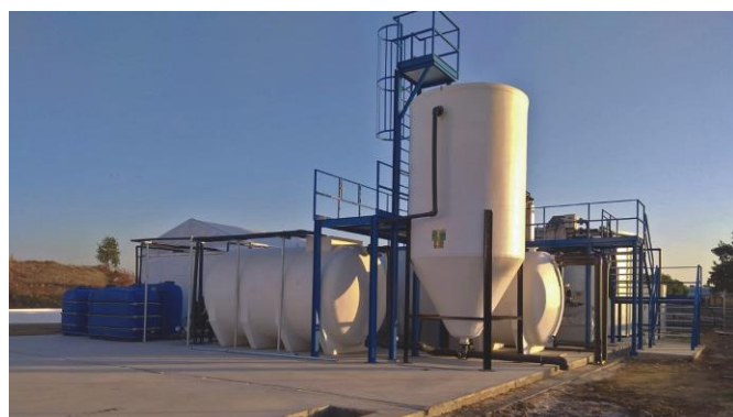
Fig. 12: Water2REturn thickener
