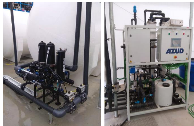
Figs. 12 & 13: Water2REturn microfiltration (left) and Ultrafiltration (right)
